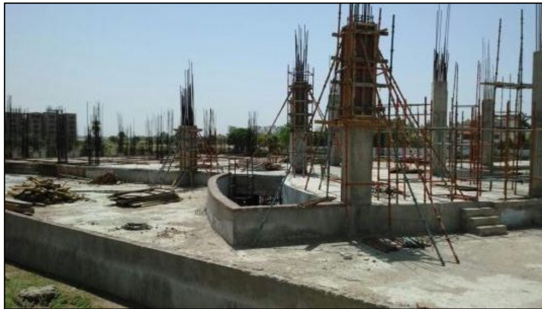
THE GREAT INDIA PLACE, Bhopal – Structure in progress
