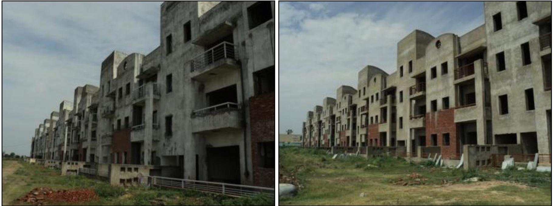
UNIHOMES, MOHALI – Structure Complete, Internal work in progress
