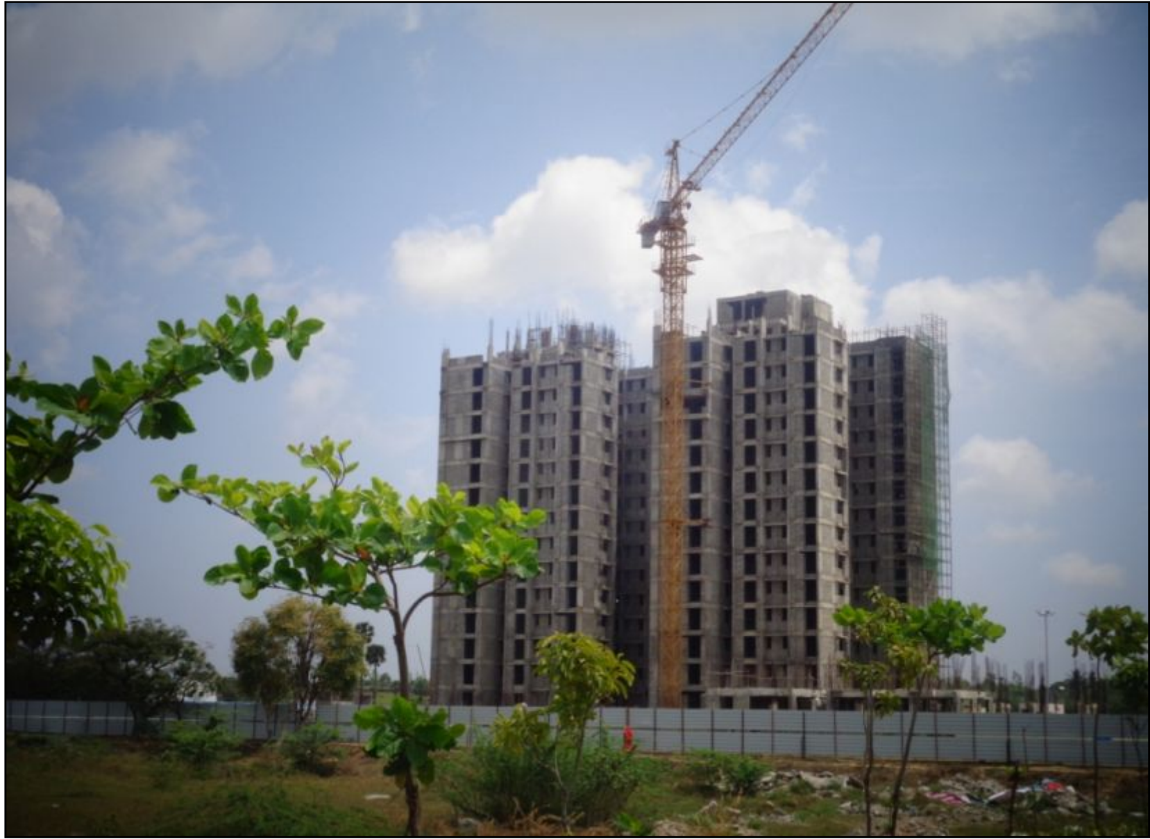
UW GARDENS, CHENNAI – Structure work in progress
