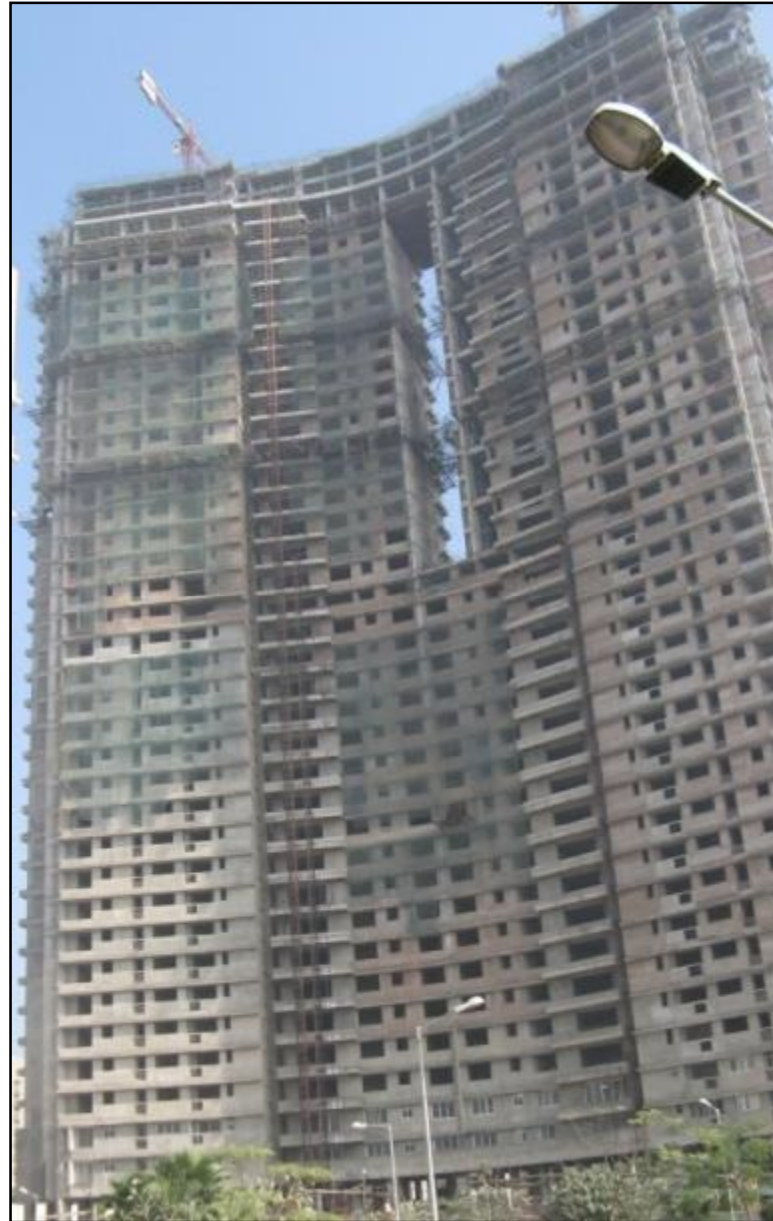
AIR, KOLKATA – Structure Complete, Internal work in progress
