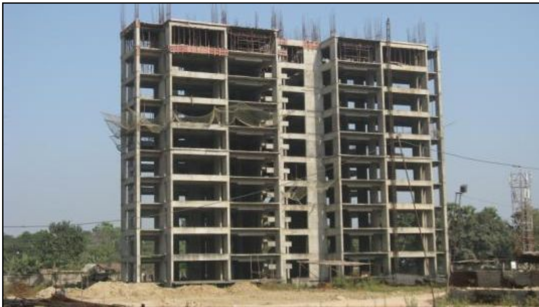
HARMONY, KOLKATA – Structure complete, internal work in progress
